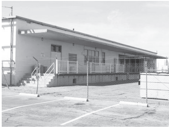
Fig. 2. China Lake Curation Facility and Archaeological Laboratory, Building 1022.
