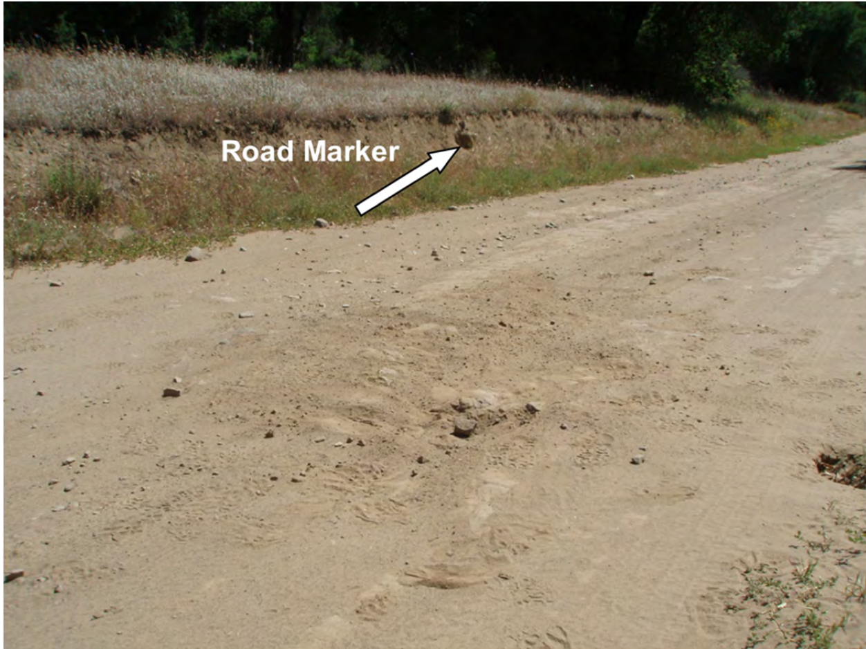
Figure 5. Road Marker on road cut face indicating road level in 1974.
