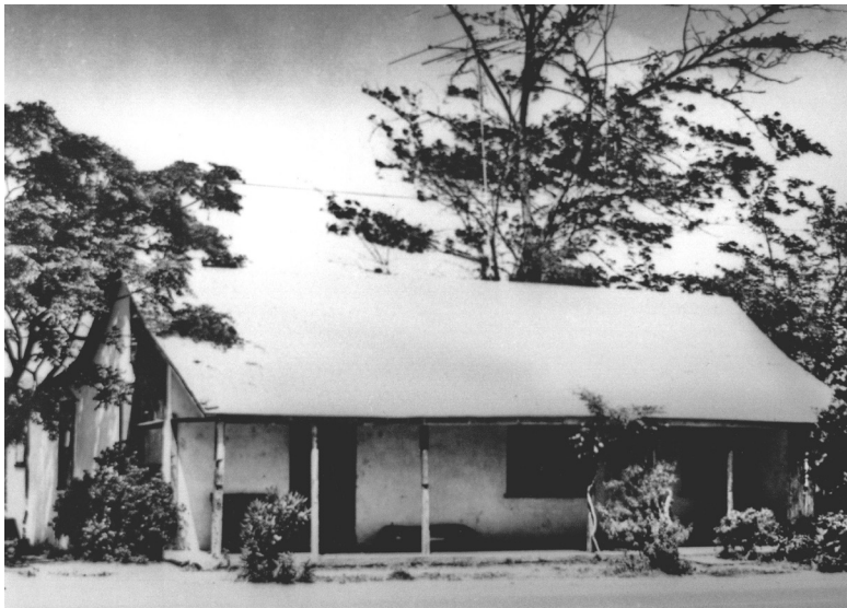
Figure 2. Silvas Adobe, Los Rios District, San Juan Capistrano. Built in 1794 by Juaneños during the construction of Mission San Juan Capistrano. Photograph courtesy of the San Juan Capistrano Historical Society.
